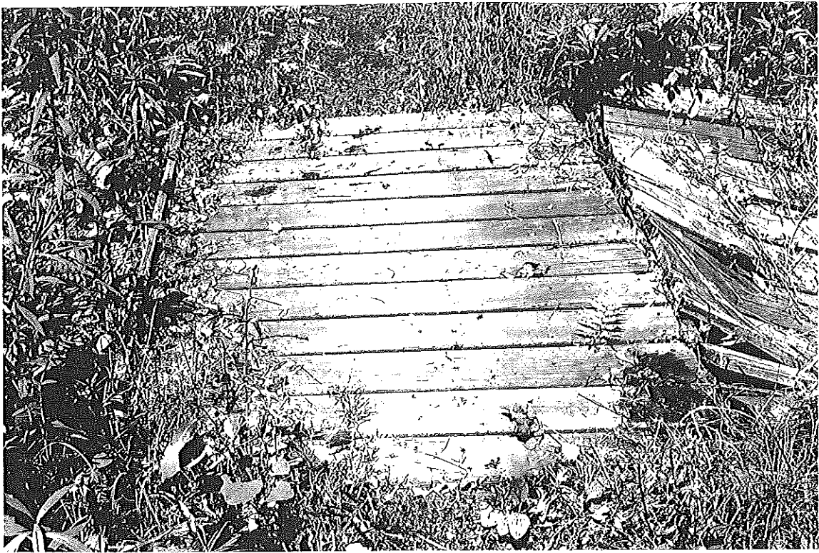
25 Main line near end of Sidewinder
